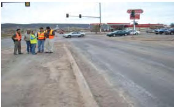
Looking north along N-12 at the intersection with N-110 (near Fort Defiance). A 62-foot urban cross-section is provided, consisting of two through lanes in each direction, with curb and gutter and turn lanes (or a raised median) at intersections.
