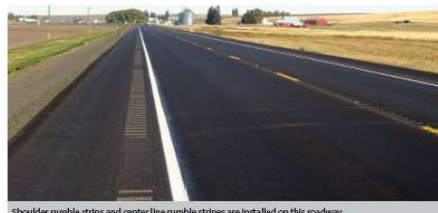
Shoulder rumble strips and center line rumble stripes are installed on this roadway.
