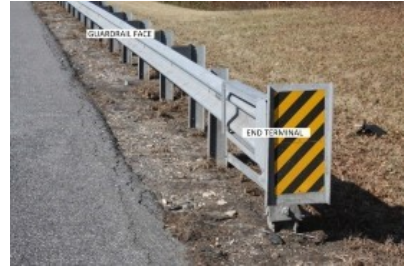
Photo Source: FHWA (2009)
