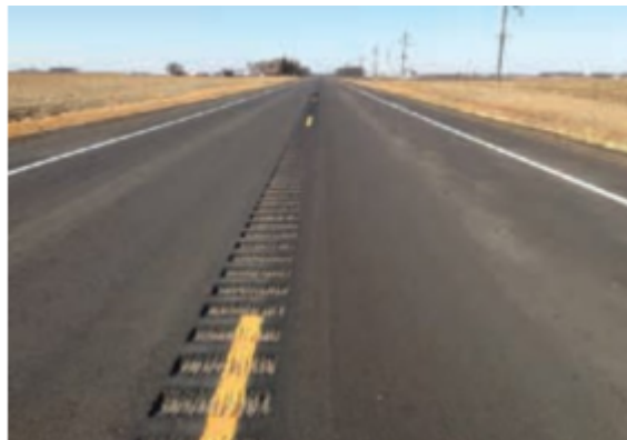
Figure 1: Sample of Installed Milled CLRS (Image: Neal Hawkins)
